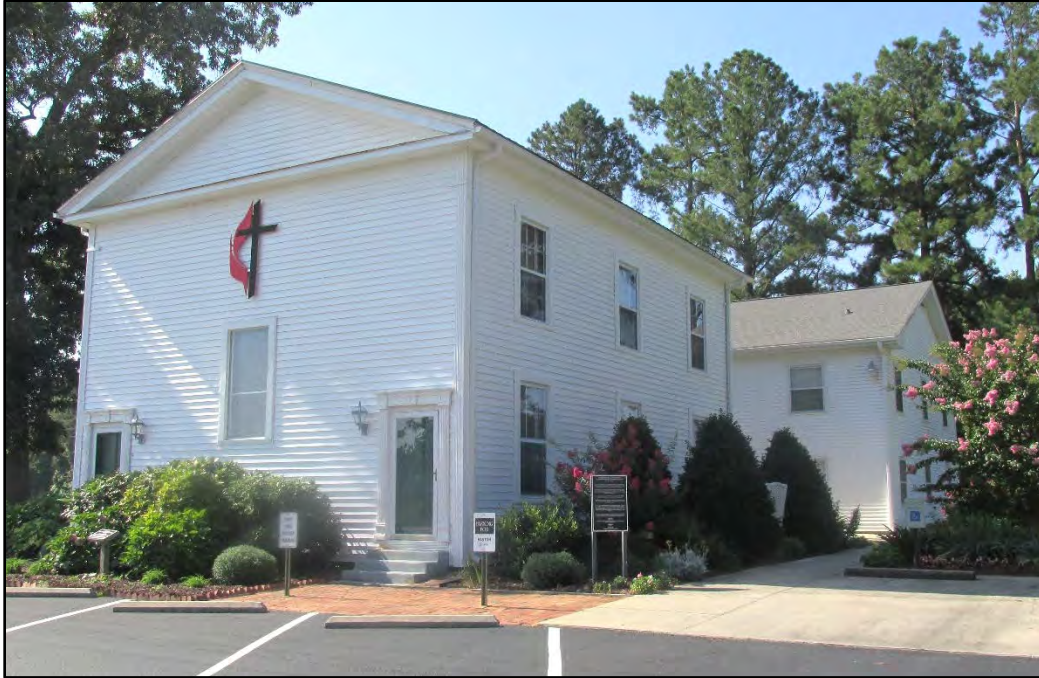
Figure 91. Elizabeth Church, north and west elevations, looking southeast.
