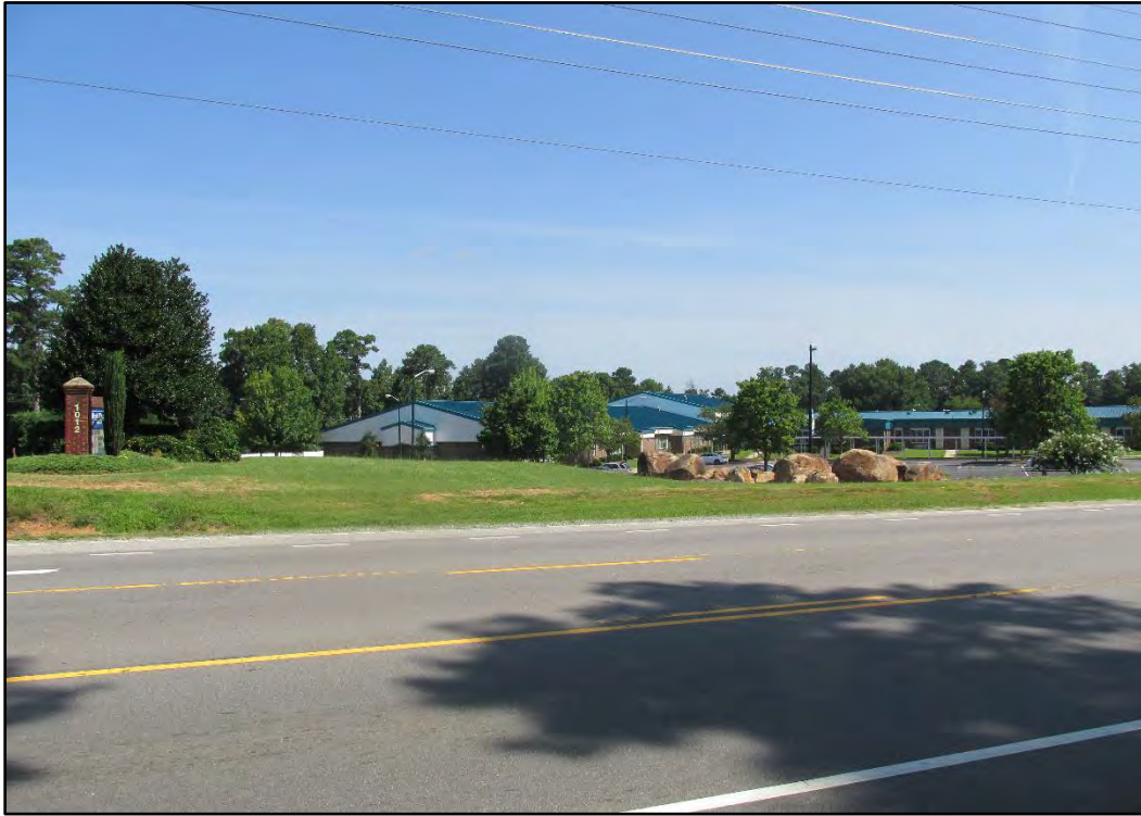
Figure 43. Looking north across NC 42 toward West Clayton Elementary School from the Keeper's House.
