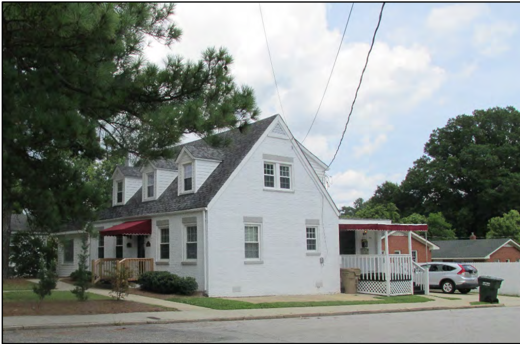
Figure 25. 425 South Lombard Street, northwest and southwest elevations.
