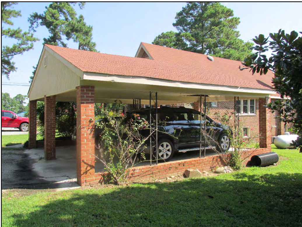
Figure 51. Carport, looking northeast.
