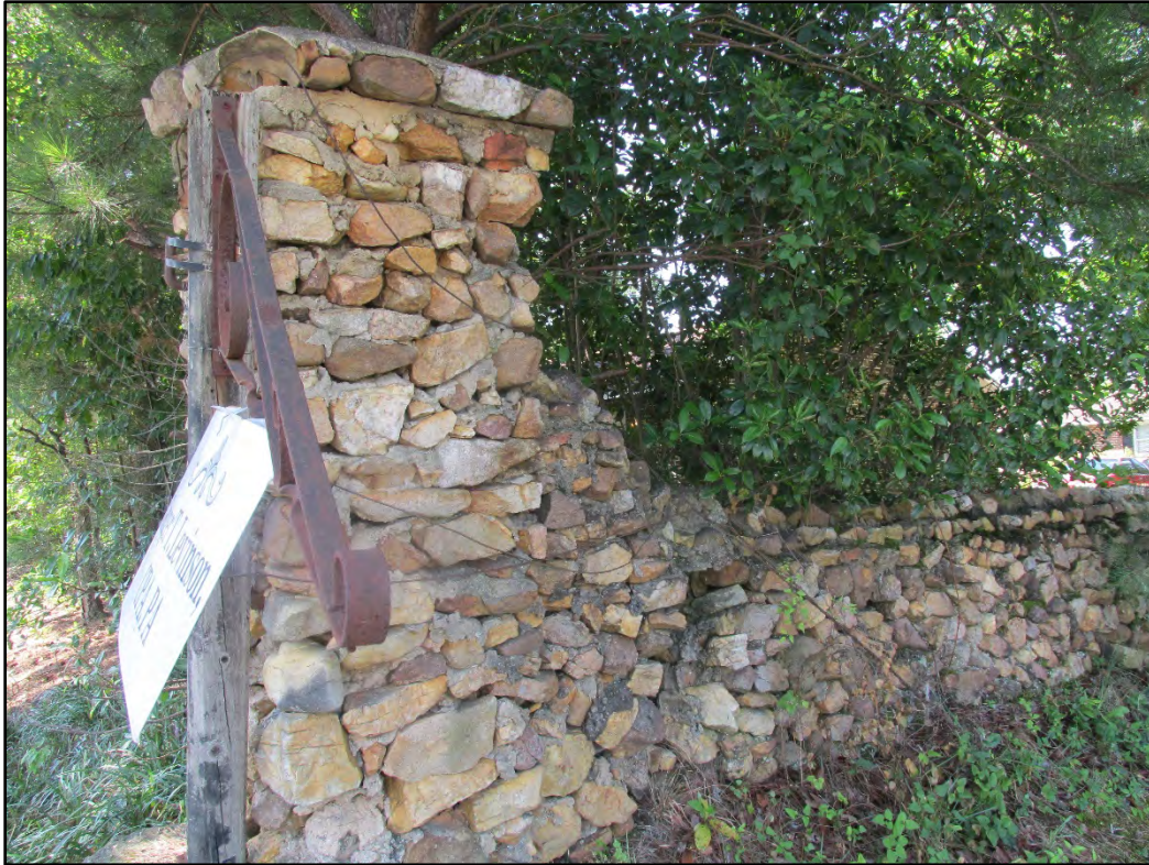
Figure 52. Stone pillar at entrance to Keeper's House, looking south from NC 42.
