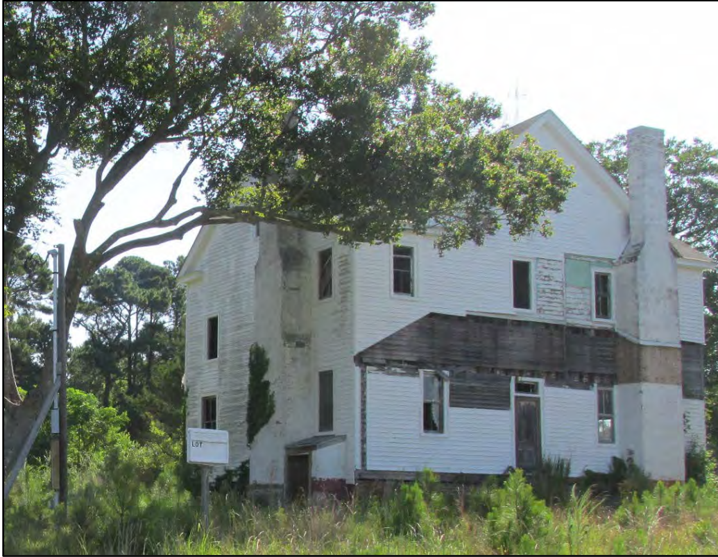
Figure 89. Sanders Family House, side and front elevations, looking northeast from Cleveland Road.
