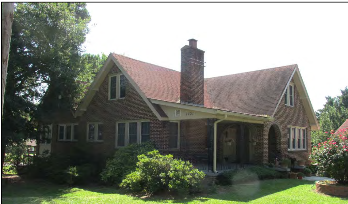
Figure 47. Keeper's House, north and west elevations, looking southeast.
