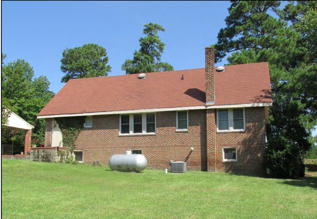
Figure 48. Keeper's House, side (south) elevation.
