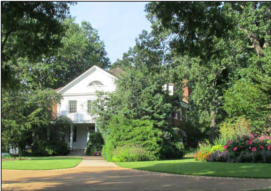
Figure 64. Garris Building façade (northeast elevation), looking south.
