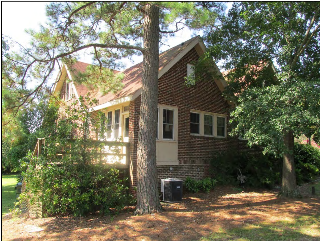
Figure 49. Keeper's House, east and north elevations, looking southwest.
