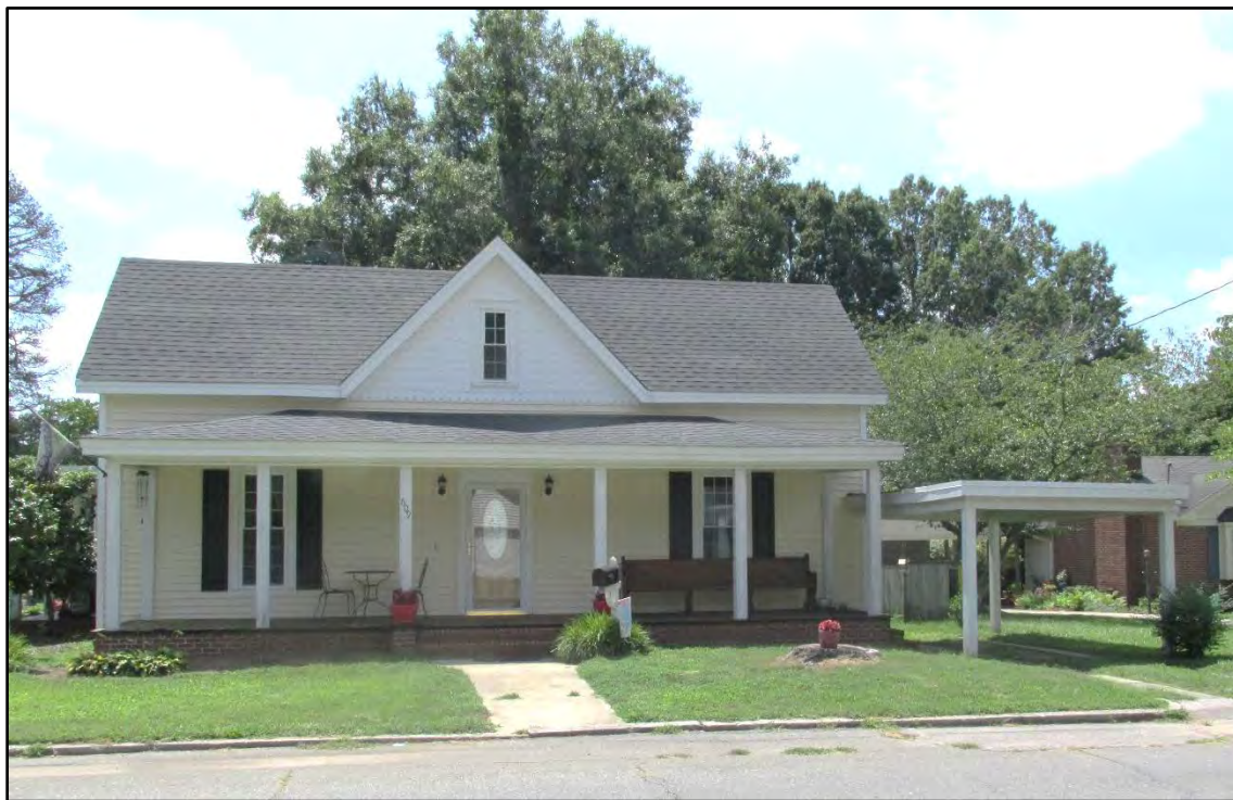
Figure 29. Example of side-gabled center-passage, single-pile house (609 South Barbour Street, northwest elevation).
