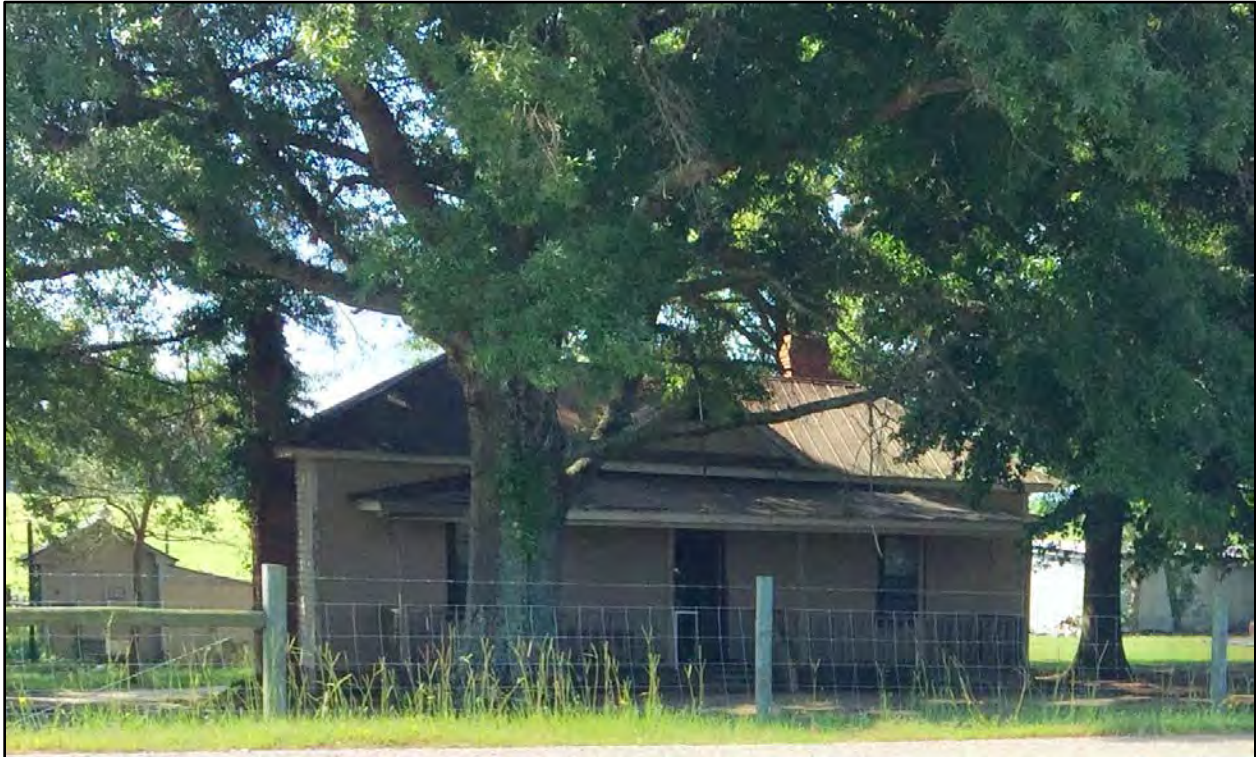
Figure 95. Lewis Jones House, front (north) elevation, looking south
