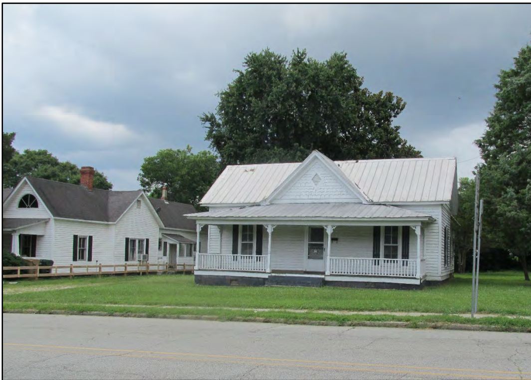
Figure 31. Façade (southeast elevation) of 502 South Lombard Street at the southwest boundary of the Clayton Historic District, looking west across the street from 501 South Lombard Street.
